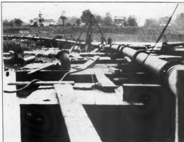
Pipe Line from Dredge to Sizing Plant
